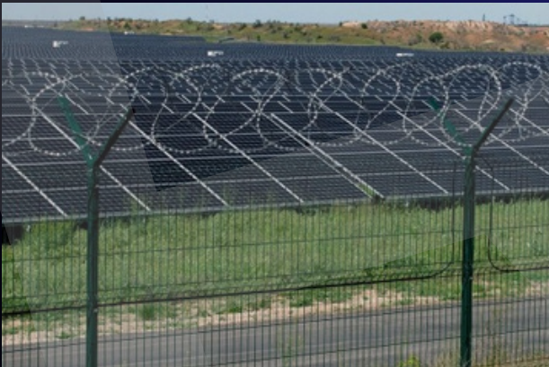
Palisade & Security fencing
